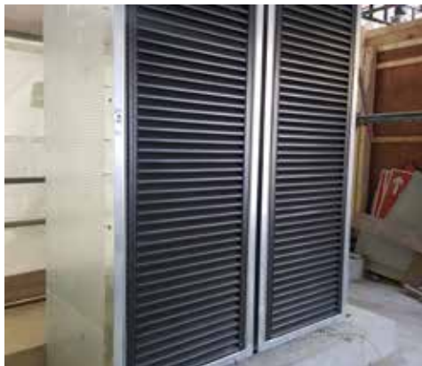
Louvre double bank joint
